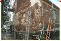
The contractors started removing the old render on Wednesday. The week was extremely hot weather and the task of removing the old render physical and dusty work. While the render crumbled easily where it had delaminated from the cob wall there were places where it was still well adhered. Progress was made on east, south and west elevations during the week. More scaffolding is required to access the wall over the kitchen roof.
