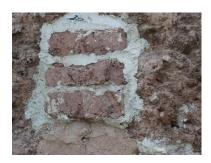
With the old render removed it exposed the cob wall. There is evidence of previous repair work to the wall where cob blocks have been added. Damaged parts of the original cob wall have been cut out and the new cob blocks fixed with lime putty.
